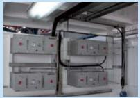
Sample Conditioning Systems (SCS) for natural gas. The SCS is installed close to the sampling point and reduces pressure from process conditions to 1-2 bar. The method of construction assures that the mercury concentration in the sample stream remains unaltered when flowing through the
