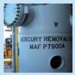
A Mercury Removal Unit (MRU) on an offshore platform. The MRU reduces the mercury in a natural gas stream via a bed of sulfurized activated carbon. The mercury concentration at the outlet is monitored to be less than 10 ng/m³; this level is regarded as harmless to plant components downstream.
